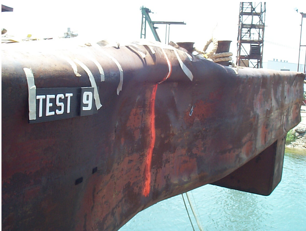
Figure F-4. Crushing damage of barge headlog, Experiment 9
