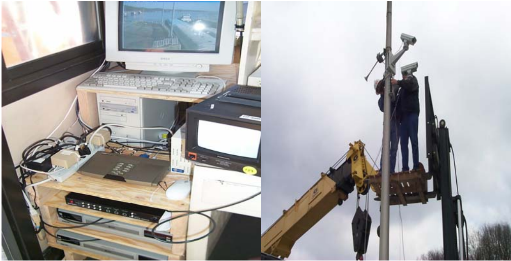
Figure B-9. Demonstration of time-lapse equipment installed at Kentucky Lock (computer acquisition system on left and time-lapse camera on right)
